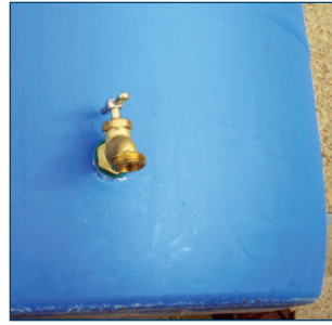
Figure 17. Hose bib facing down.
